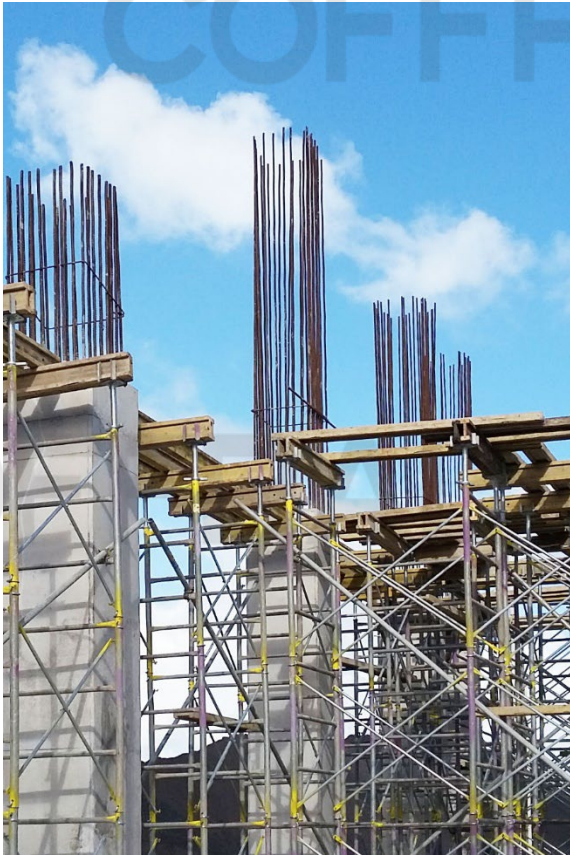
Staflex Concrete Slab Shoring
