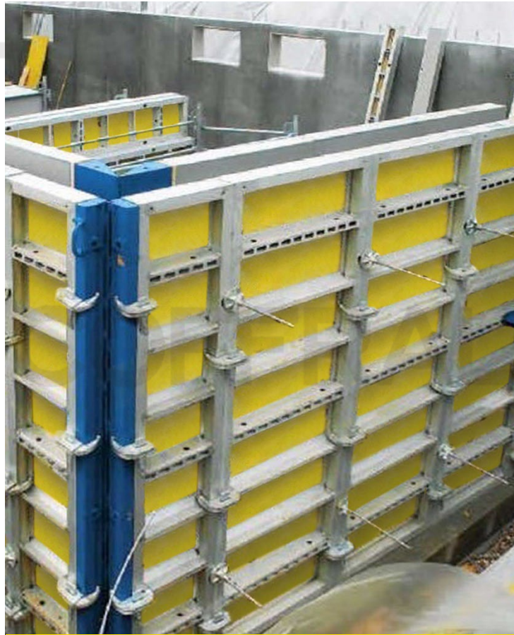
Wall Formwork
