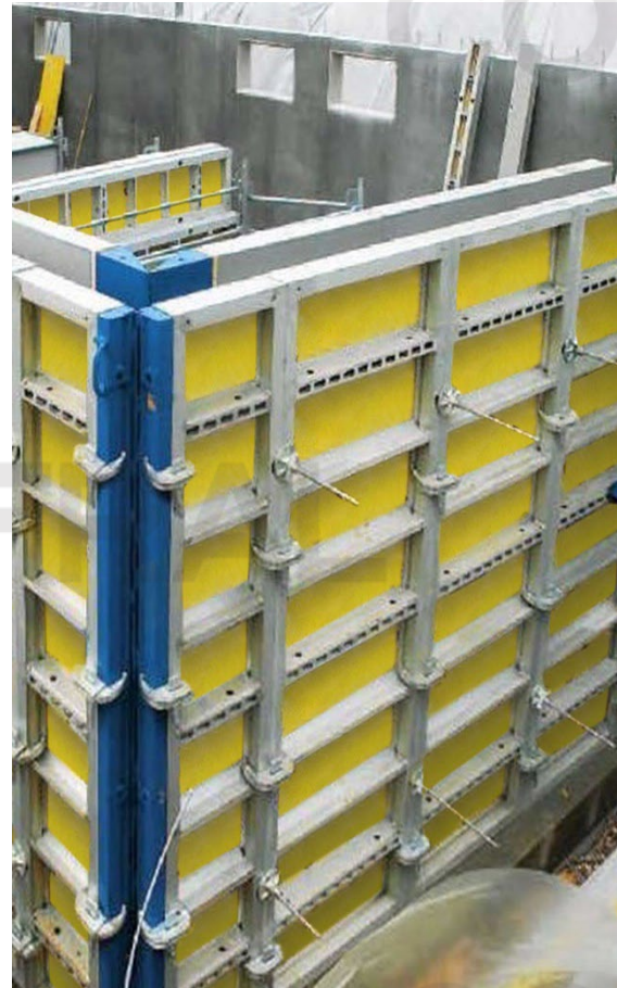
Vertical Formworks
